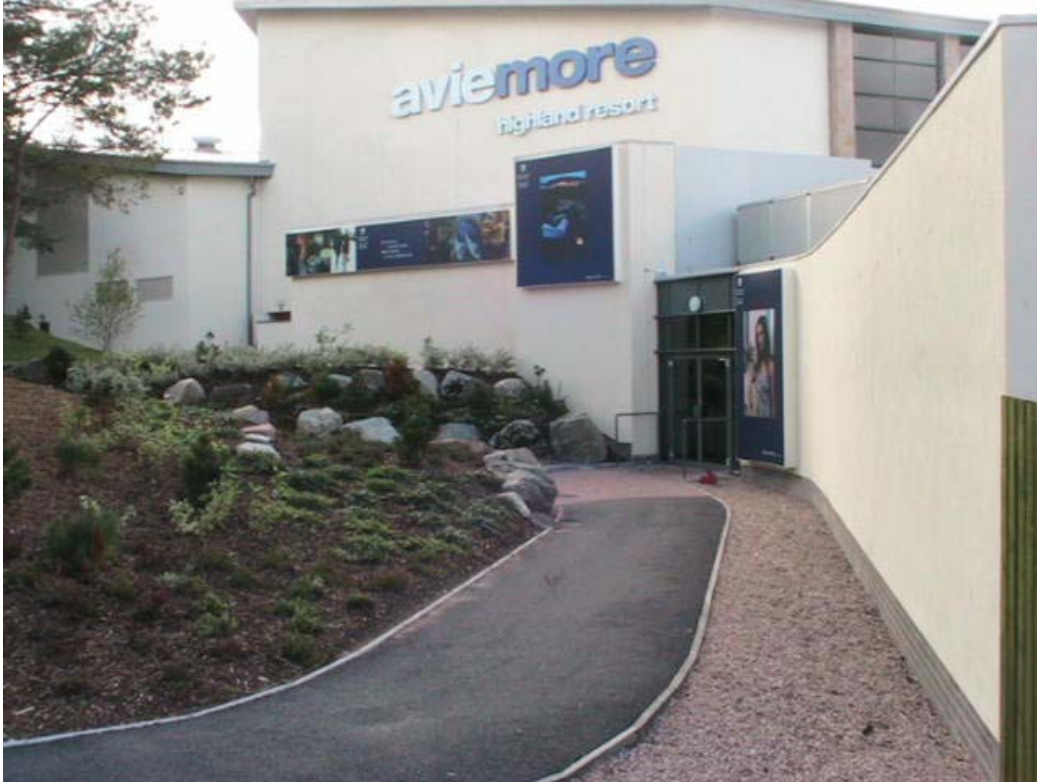
Fig. 2 Eastern entrance signs, the 3 lower level panel signs are the subject of this application.
